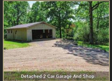
Detached 2 Car Garage And Shop
